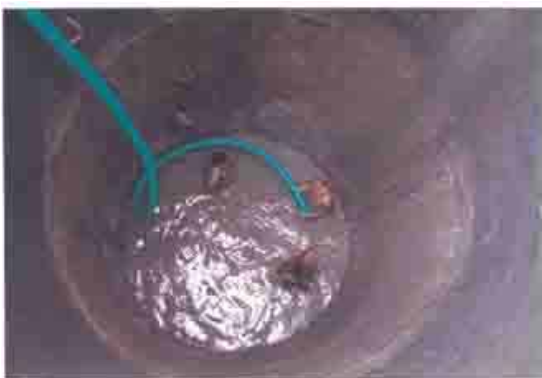
Figure 9(a): Cleaning of the dug-well
