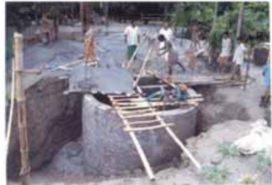
Figure 10(b): First stage of construction
