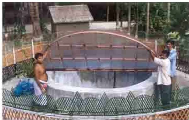
Figure 9(b): Use of glass fibre sheet to prevent surface contamination
