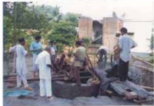
Figure 10(c): Second stage of construction
