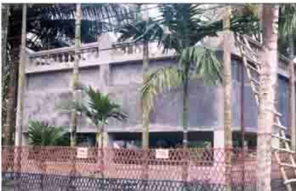
Figure 9(c): The two storied storage tank.
